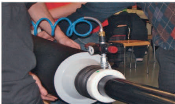
Fig. 1: installation with gas cushion method
