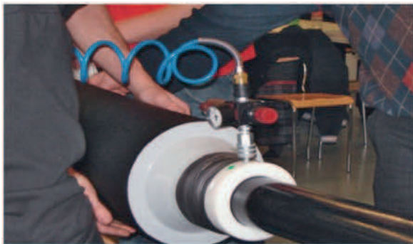
Fig. 1: installation with gas cushion method
