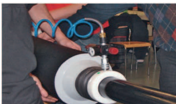
Fig. 1: installation with gas cushion method
